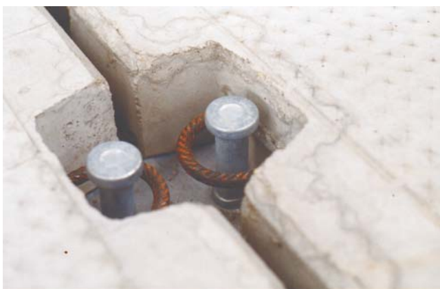
Figure 5: Joint between two ceiling slabs in a multi-storey car park, before pouring the mortar
