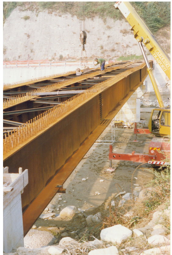
Figure 13: Composite bridge made of I-beams during assembly
