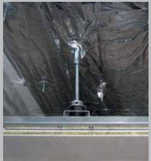
Welding elements for ceiling suspensions
